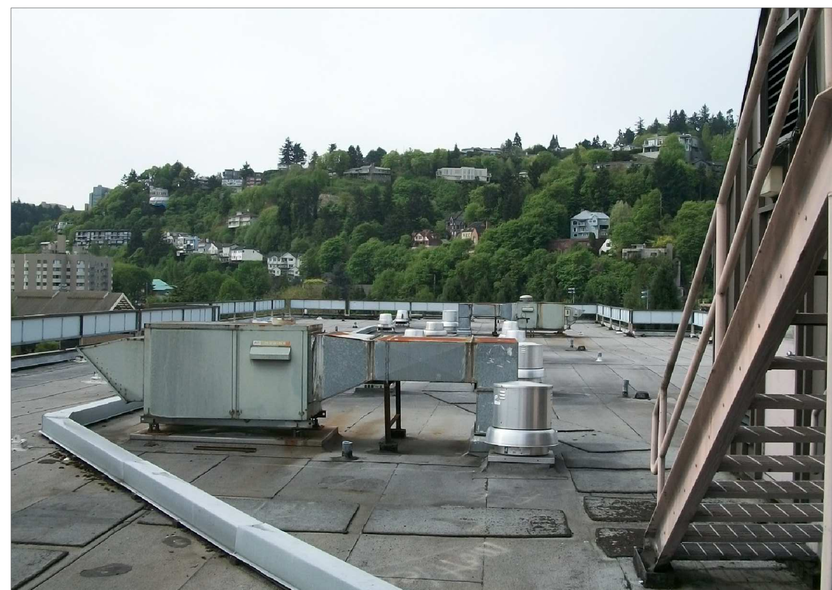
Existing Roof View
