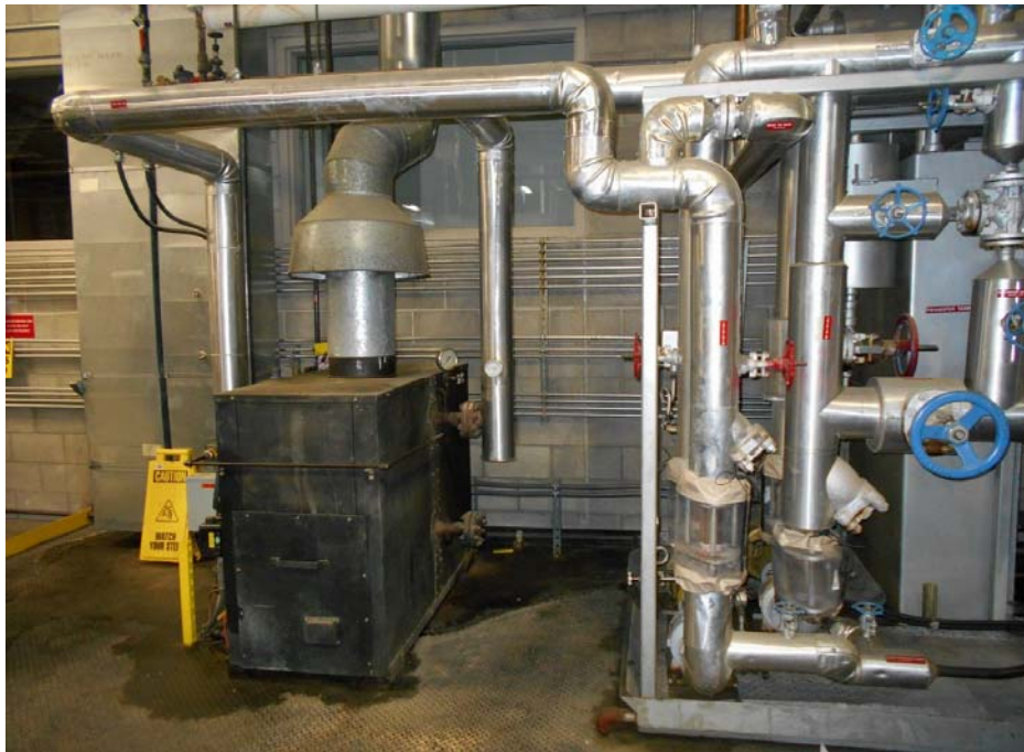
Press steam piping/valve pallet approximate shipping dimensions; 8' x 6' x 6', 2,500#
