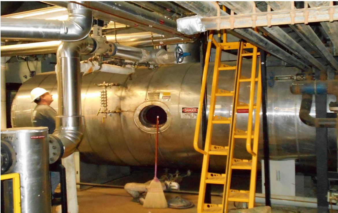
Press steam accumulator approximate shipping dimensions; 8' x 8' x 20', 10,500#
