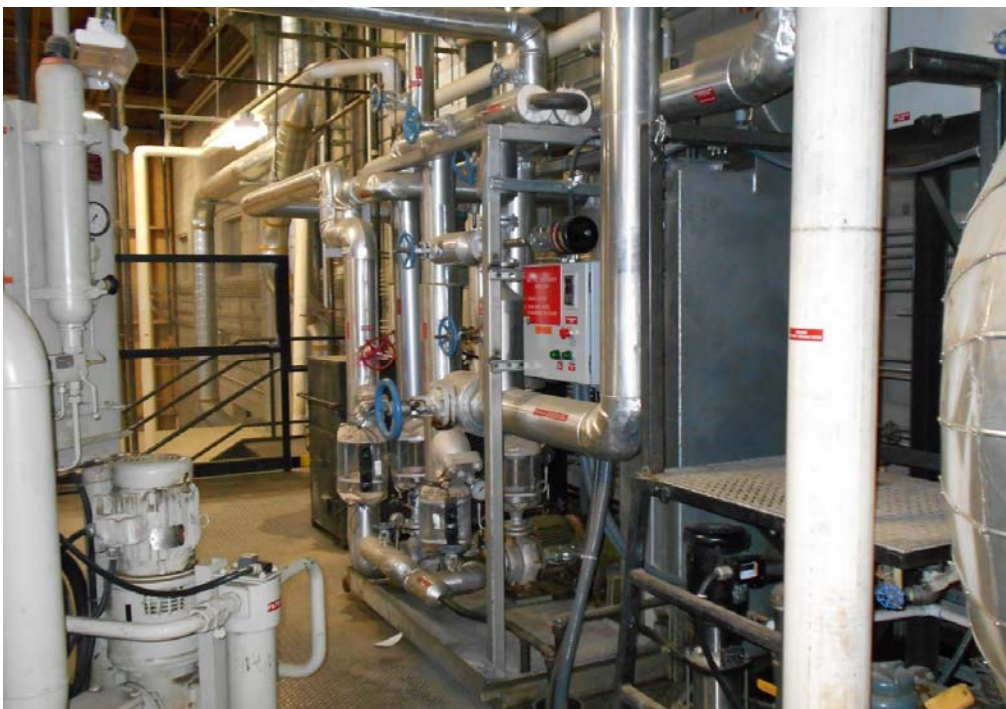
Press steam piping/feedwater assembly approximate shipping dimensions; 6' x 6' x 10', 2,500#
