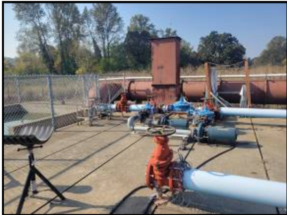
Existing Piping and Pumps to be Removed at Exterior Test Slab Area
