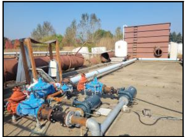
Existing Piping and Pumps to be Removed at Exterior Test Slab Area. Existing Above Ground Storage Tank Can be Seen.
