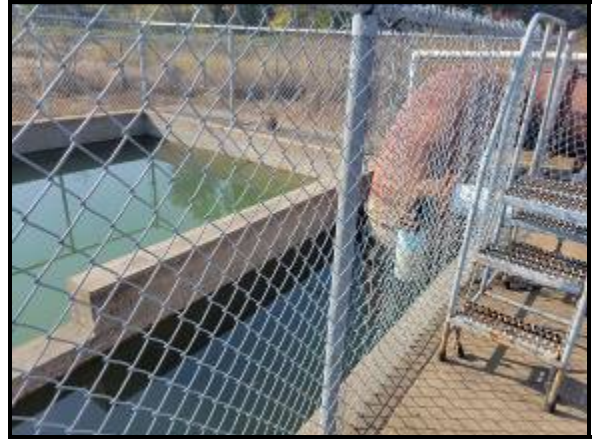
Location for New Drainage Sump Pump in Existing Sump Pit Well
