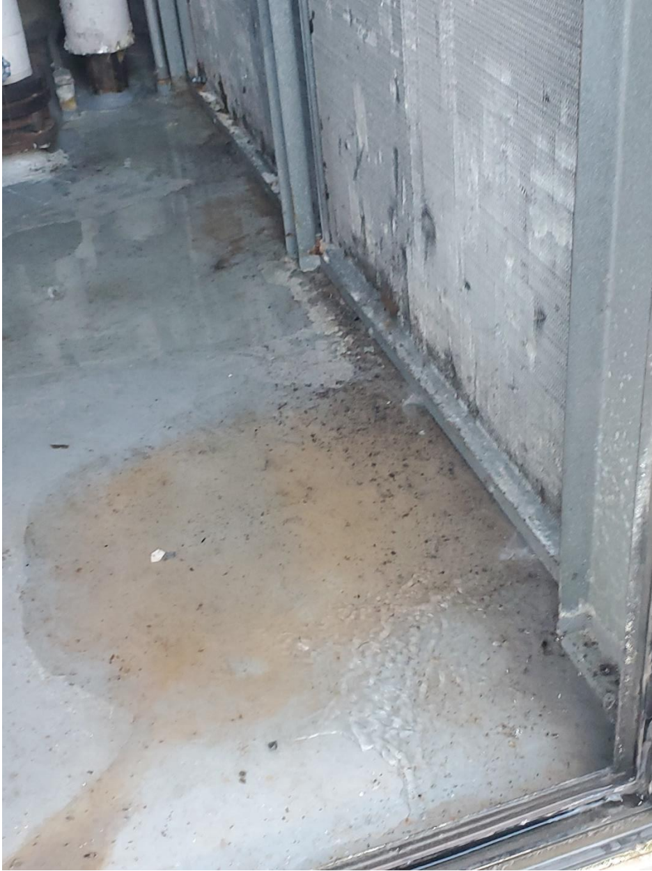
Photo 3: AHU-1 Heat Recovery Coil Plenum
