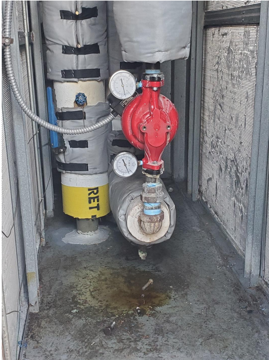
Photo 4: AHU-1 Heating Coil Plenum
