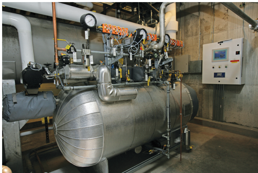
FIGURE 6. Liquid Effluent Sterilizer*
