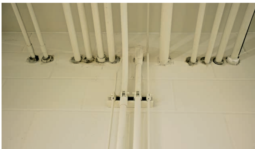
FIGURE 18. Caulking around Service Intrusions*
