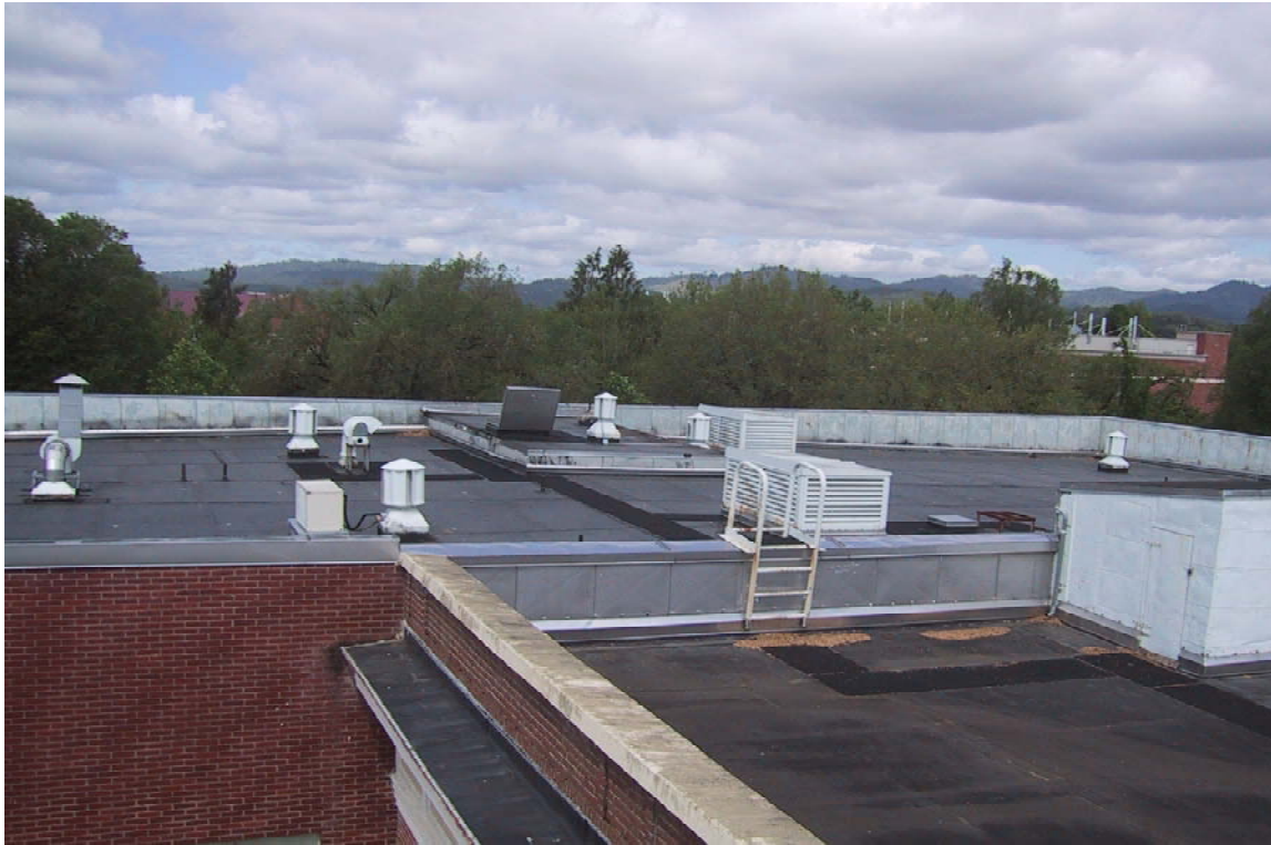
Roof Areas "C & D"
