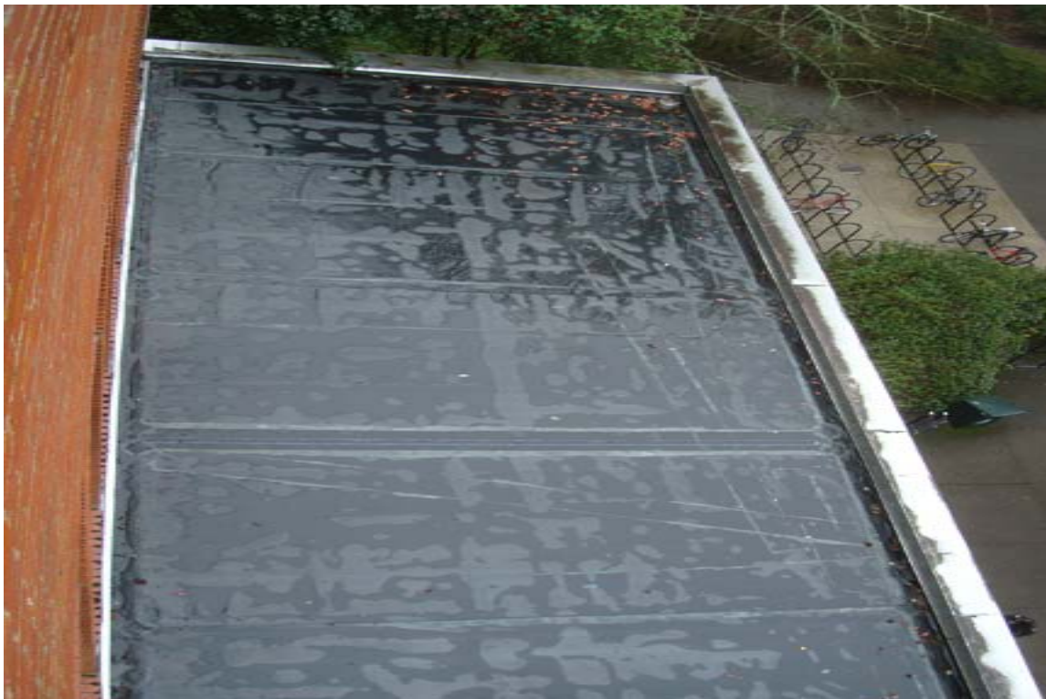
Roof Area "F" recently replaced.
