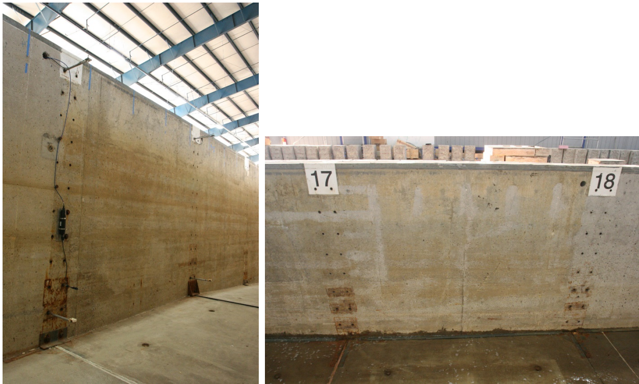
Figure 10. Sample images of the bolt-hole pattern in the Large Wave Flume.
