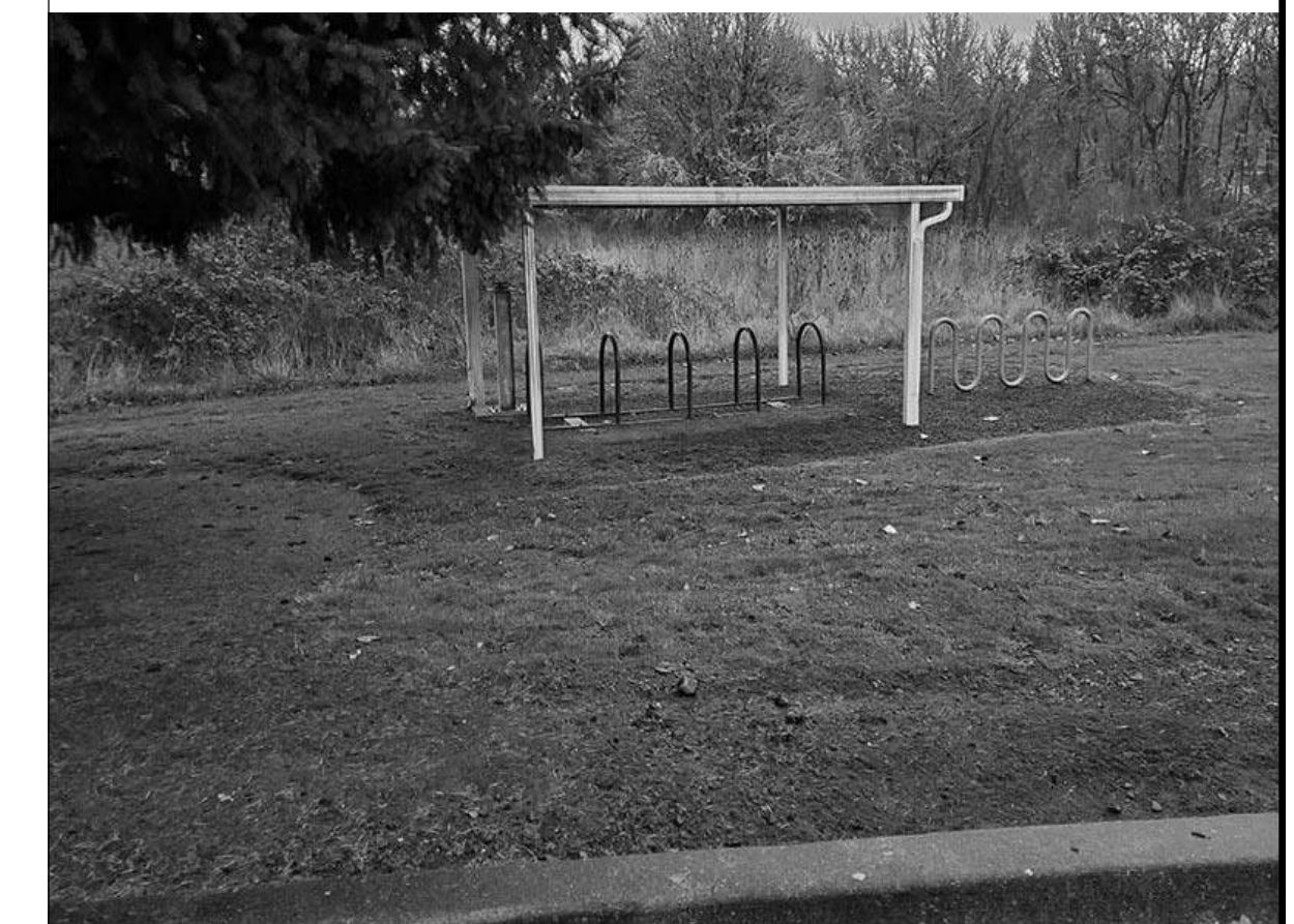
EXISTING COVERED BIKE RACKS. (S) U RACKS, (1) RIBBON (NOT INCLUDED IN BIKE PARKING COUNT)
