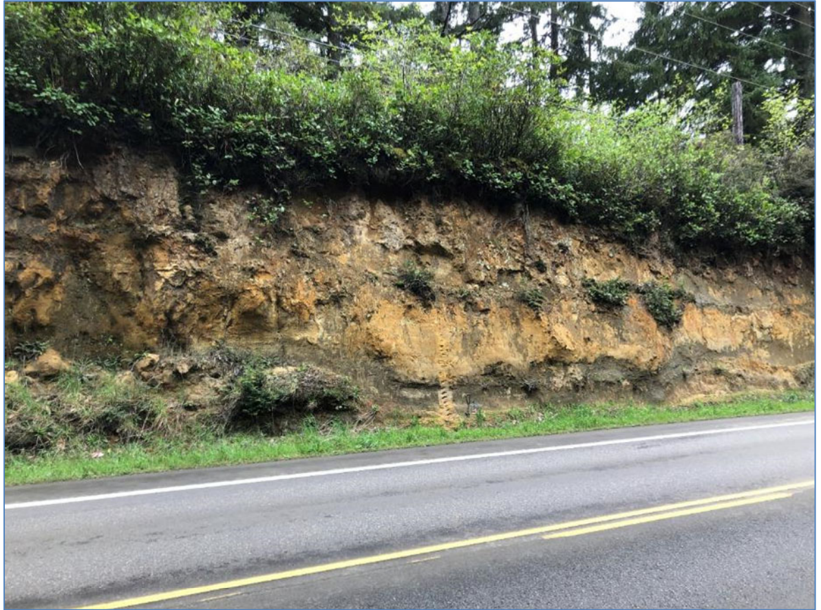
Photograph 3. These terrace deposits are exposed along US101 south of the HDD alignment. This cut is nearly 20 feet high and subvertical.
