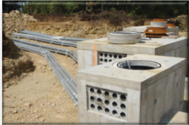
Figure 12 - Typical Beach Manhole, for illustrative purposes only
