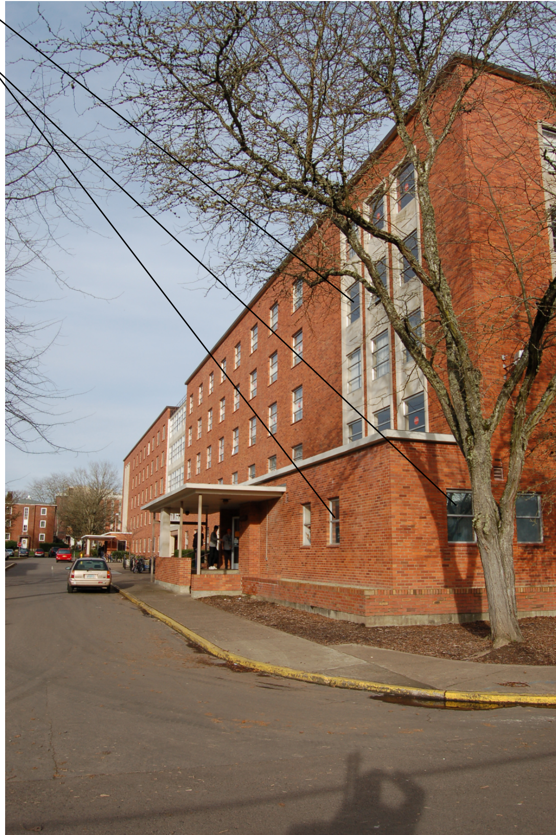
existing window conditions
