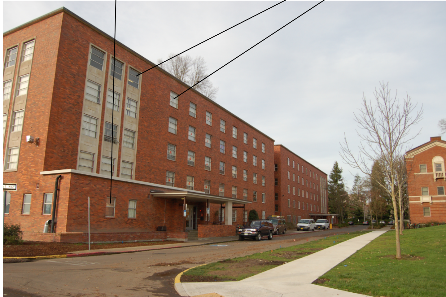
existing window conditions
