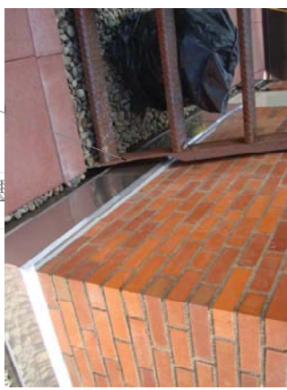
6 PENTHOUSE DOOR THRESHOLD AS.2 1" = 1'-0"
