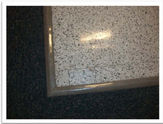
Sample 14-072A.9, Floor Tile (Top), Non-ACM Sample 14-072A.10, Gray Floor (2 nd ), Non-ACM
