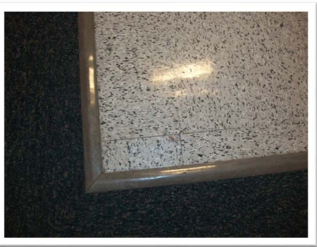
Sample 14-072A.9, Floor Tile (Top), Non-ACM Sample 14-072A.10, Gray Floor (2 nd ), Non-ACM
