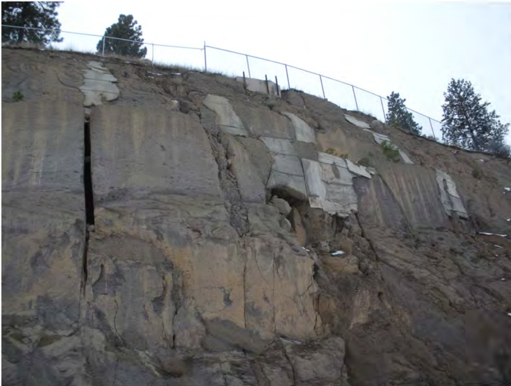
Photograph 13: Showing extensive jointing and concrete patching.
