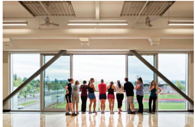
Exterior sliding glass door systems and ceiling fans introduce natural ventilation in spaces such as a multi-purpose room
