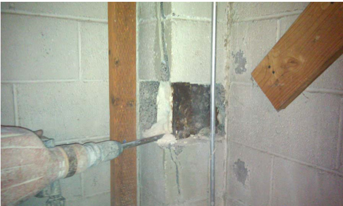
Figure 4: Corroded Steel Column within Pilaster
