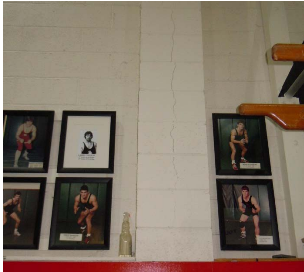
Figure 3.14 – 2 nd Column North of Southwest Corner
