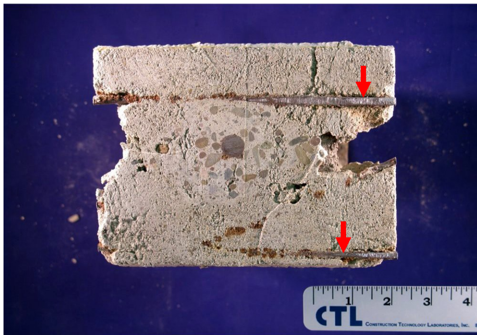
1d. Bottom surface showing a steel wire tie (arrows) partially embedded in joint mortar. The tie exhibits brown surface rusting.
