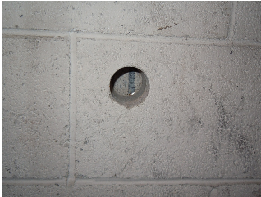
Figure 3.10 – Vertical Rebar in Boiler Room
