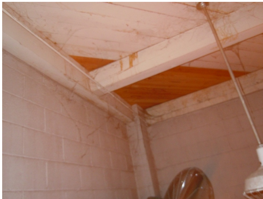
Figure 3.3 – Southwest Corner of Storage Room Roof
