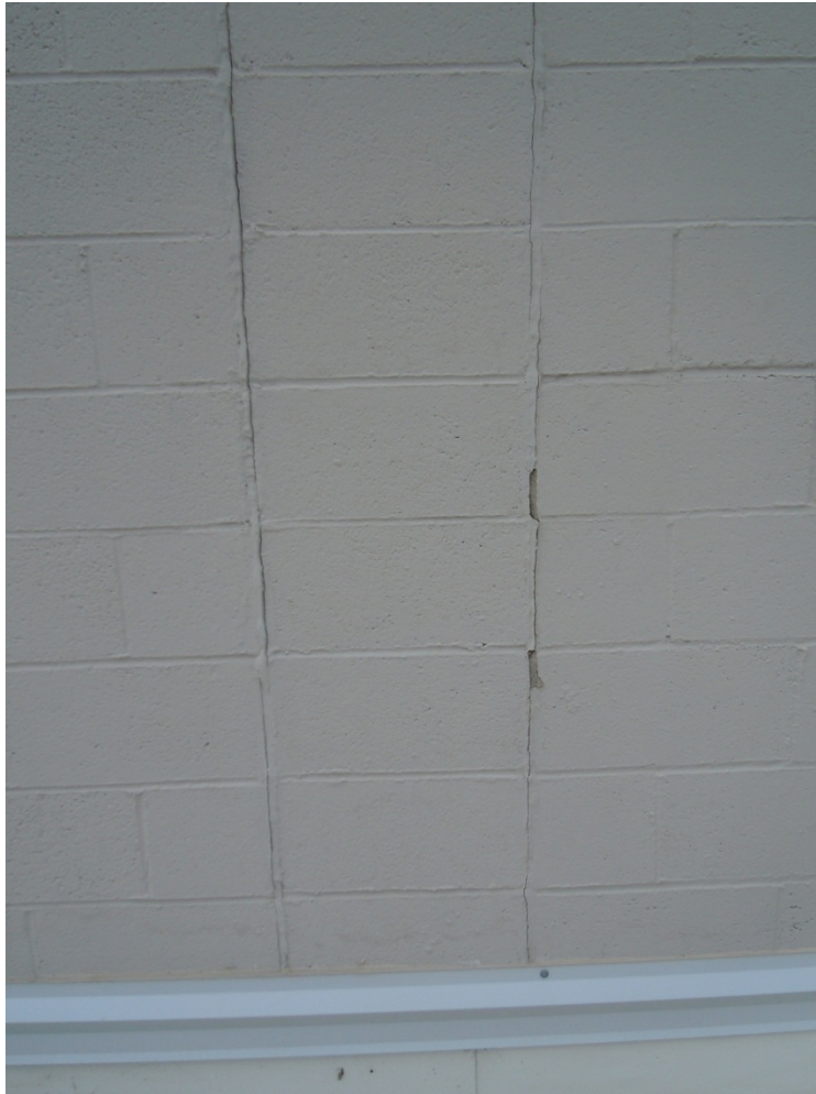
Figure 3.7 – Expansion Joint at Each Side of Masonry Pier
