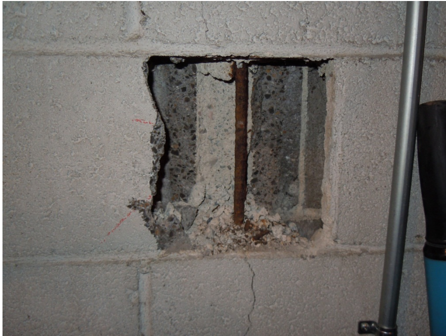
Figure 3.8 – Vertical Rebar in Storage Room
