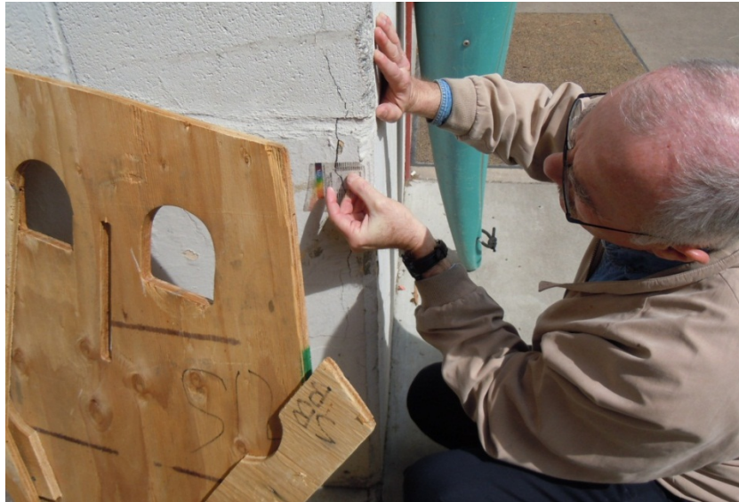
Figure 3.2 – Southwest Corner of Storage Room
