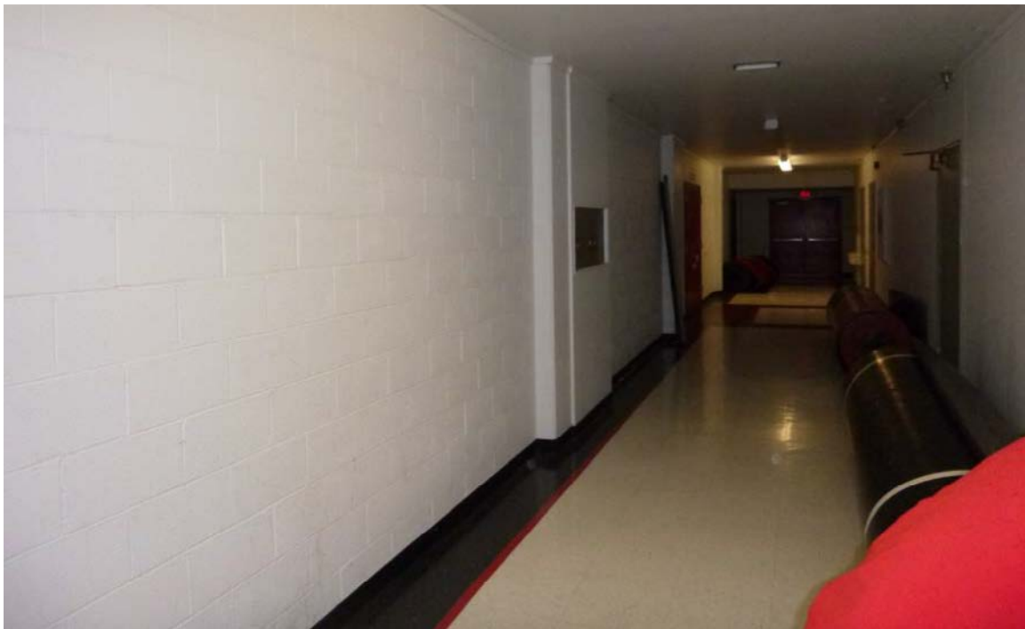
Figure 6: Interior Wall Condition
