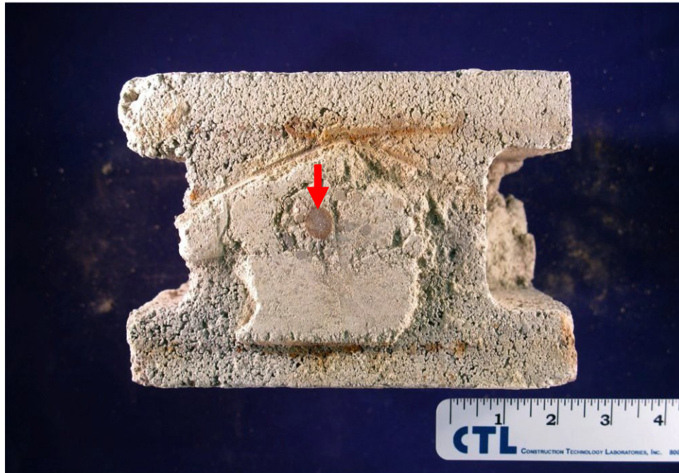
2c. Top surface, locally covered with joint mortar. Arrow designates a reinforcing steel bar. The rebar exhibits no visible corrosion.
