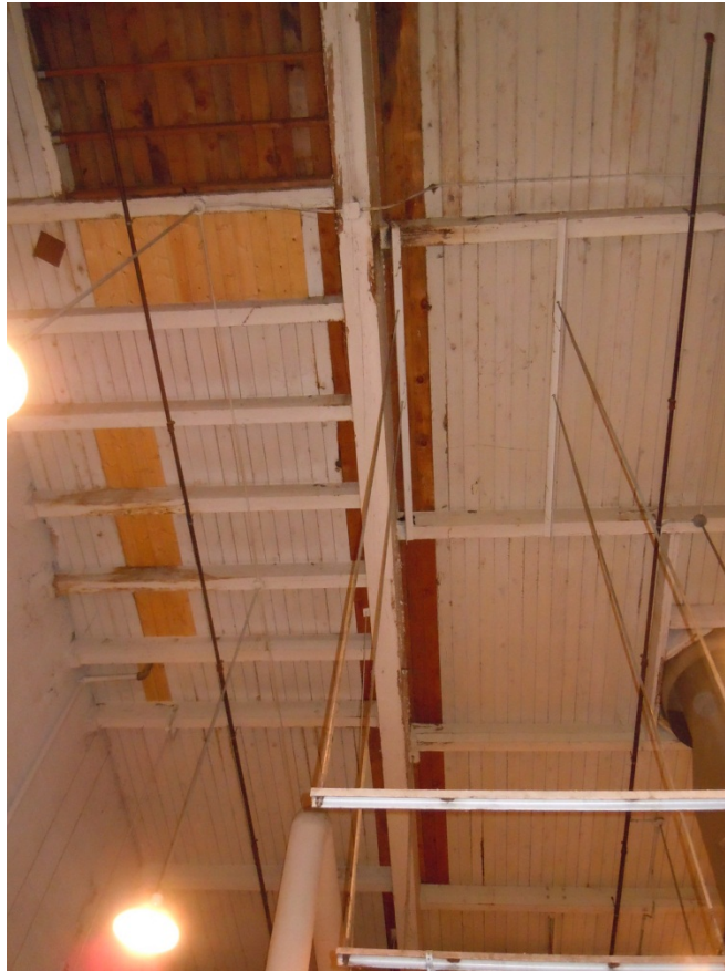
Figure 3.16 – Boiler Room Roof Sheathing
