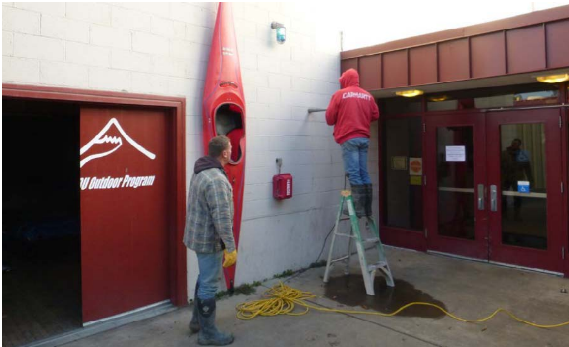
Figure 8: 2" Core Sample at South West Wall
