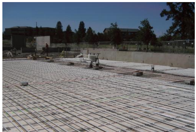
Tubes being laid out for radiant slab system
