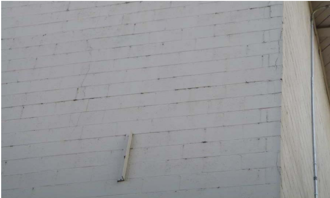
Figure 5: North West Exterior Wall Condition
