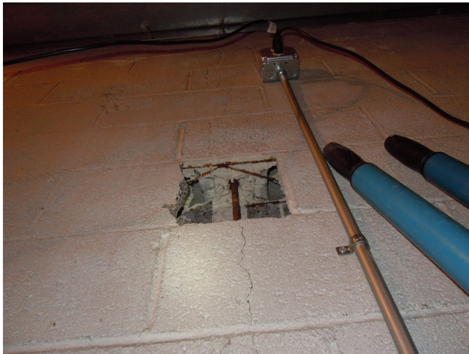
Figure 3.9 – Horizontal K-web Reinforcing in Storage Room
