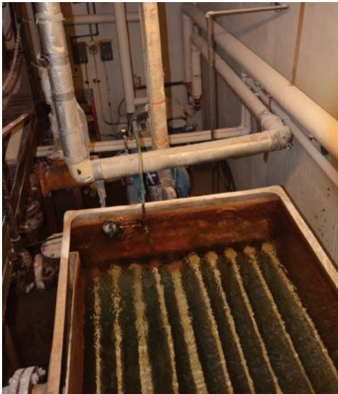
Multiple pieces of McNeal's equipment, such as the pool filtration system, are at either the end of or past their useful life.
