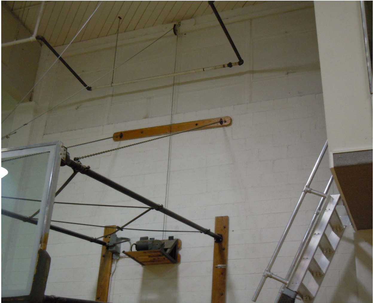
Figure 3.19 – Diagonal Cracks at Basketball Hoop
