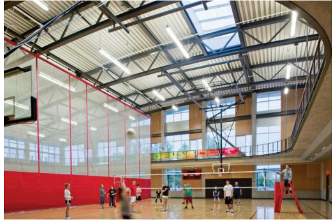
A structural roof system of steel trusses were used to span the gym at Western Oregon University.
