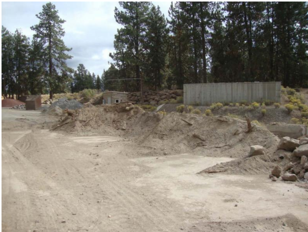
PHOTO 8: View of the former scale house area located in the eastern portion of the subject property . Note the soil mounds with organics, rocks, and concrete in the foreground and the cistern to the right.
