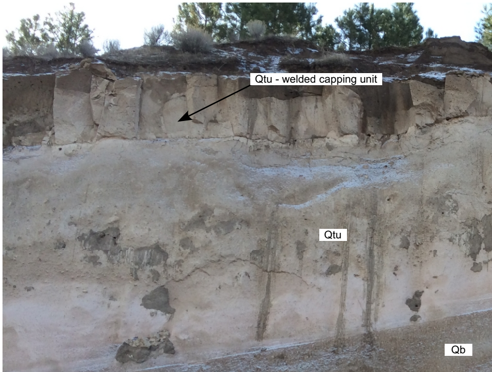
Photograph 3: Example of Qtu and columnar jointed, welded tuff capping unit.
