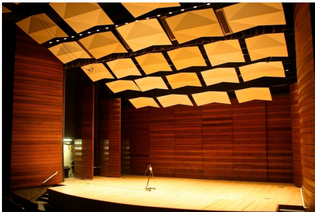
Rotating Panels Near Pinrail to Remain
