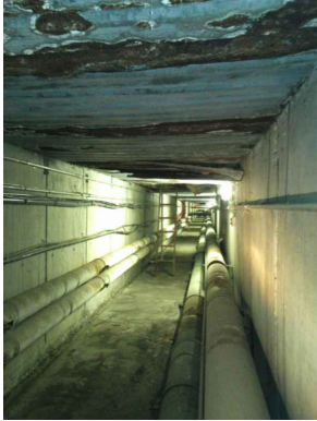
1 ROOF CORROSION
