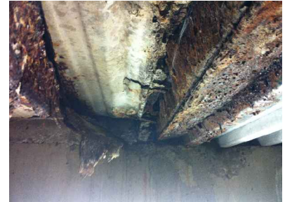
5 LOCALIZED CORROSION ± AT FIRE ACCESS
