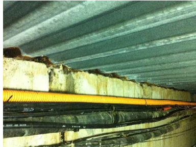
5 END PANEL CORROSION ± AT FIRE ACCESS
