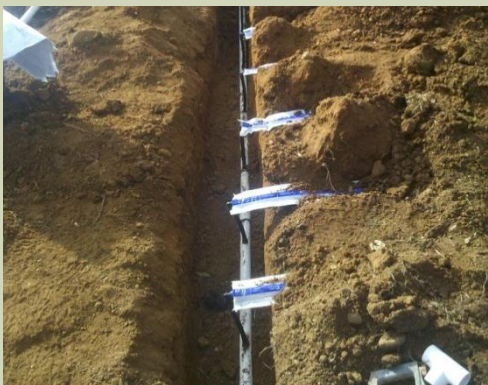
Figure 4.1.1: A header pipe installed at a depth of 8 inches
