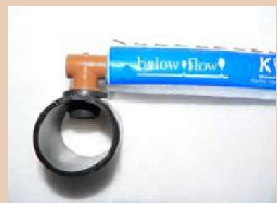
Figure 5.5.3: Pull KISSS BFW material up, covering fitting.
