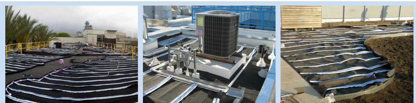
Figure 8.1.1: KISSS laid out and connected to headers and footers on-grade.
