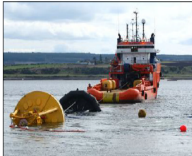
Figure 1. Ocean Power Technologies PB150 being deployed in Scotland. A similar device is planned for deployment in Oregon in 2012.
