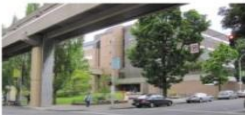
Site from Northwest
