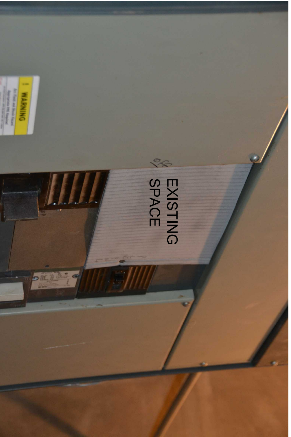
PROVIDE NEW 225/3 IN EXISTING SPACE. MATCH EXISTING.
