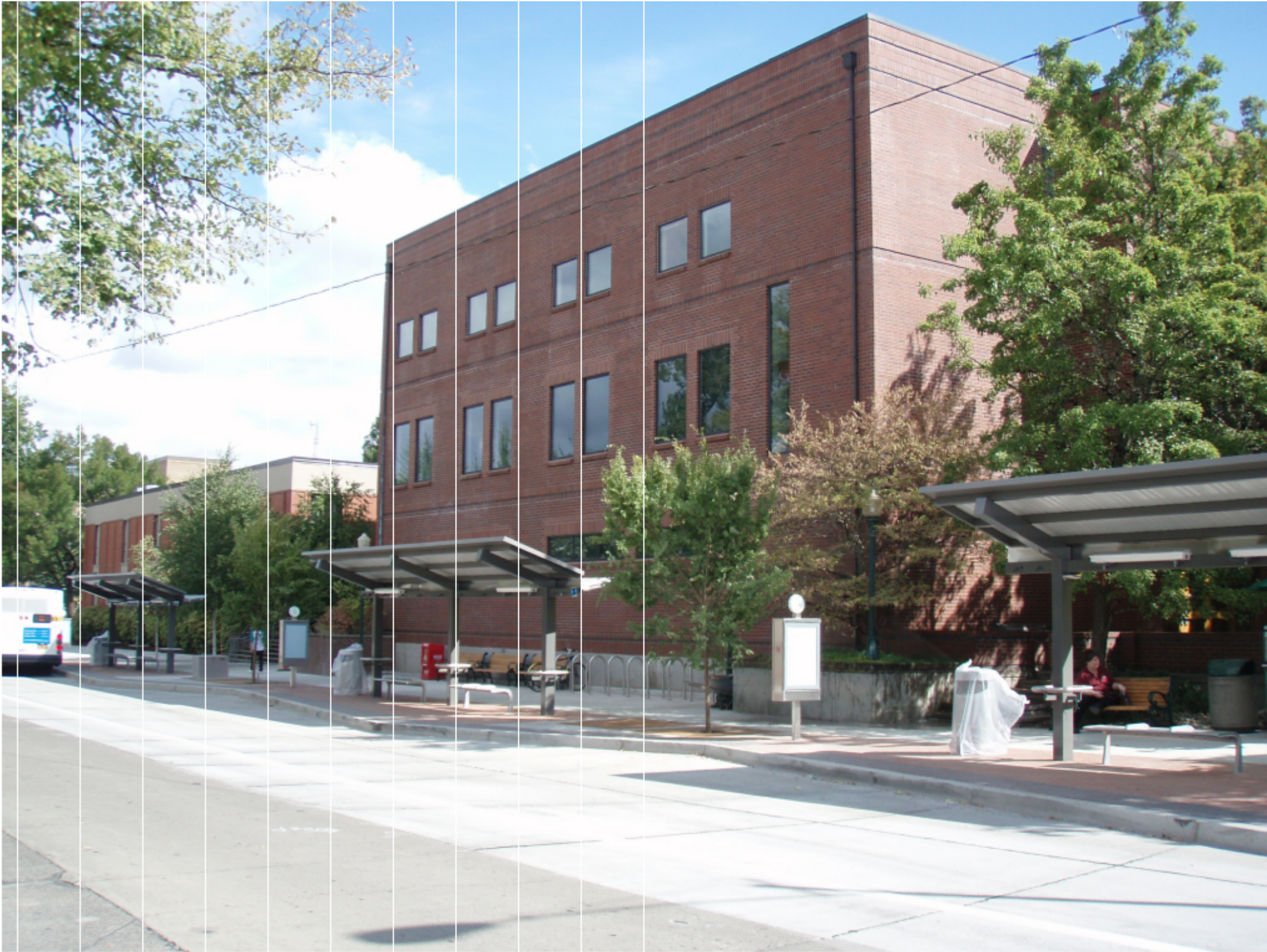
THE CHILES CENTER - WEST ELEVATION
