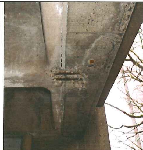
Waffle joists at fourth floor north elevation
