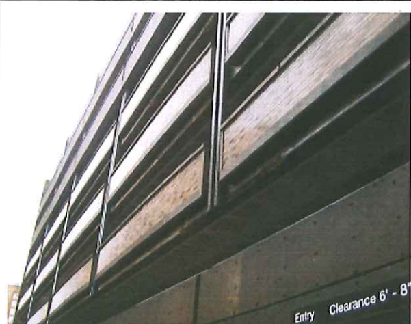
East Elevation, perimeter beam concrete removal at several locations
