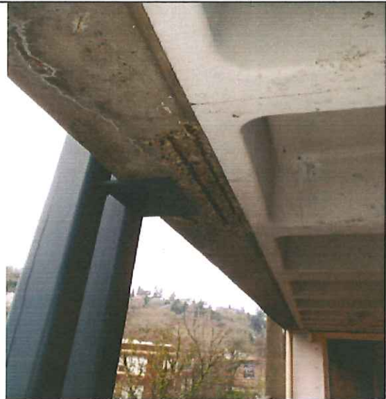
West elevation, sixth floor
