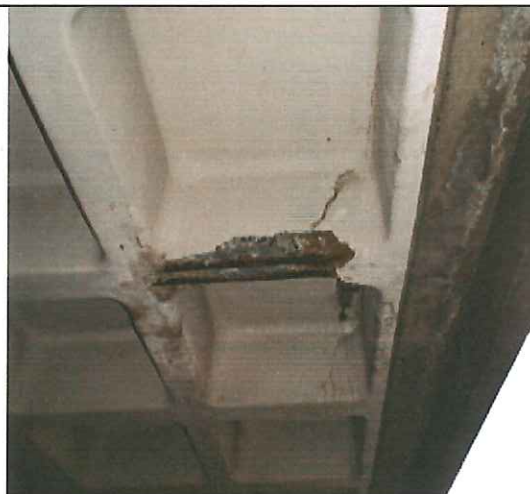
Waffle joists at fifth floor north elevation
