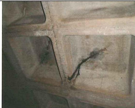
Waffle at fourth floor slab
