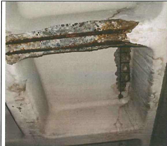
Waffle at Sixth floor slab, north elevation
