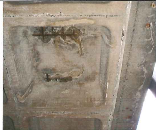
Waffle at fifth floor slab, west elevation
