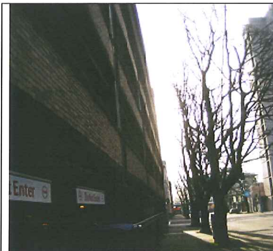
East Elevation, bowed precast panels
