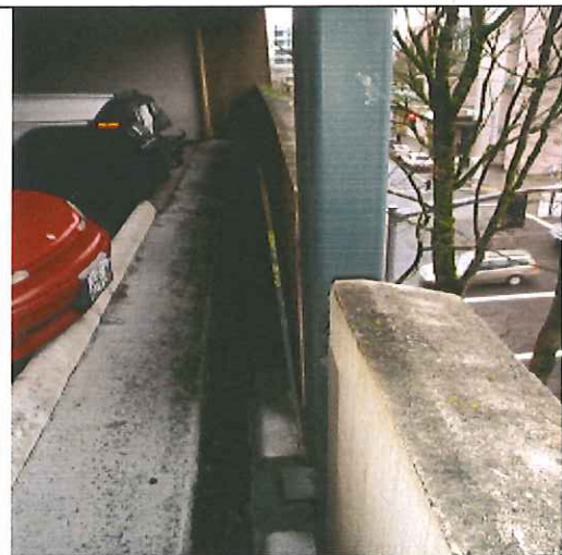
South Elevation, bowed panel at fifth floor east end
